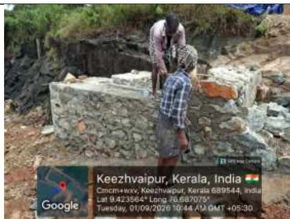
Figure 7: Photographs of garland drains and silt traps under construction
