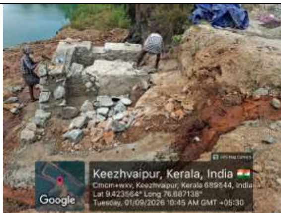
Figure 7: Photographs of garland drains and silt traps under construction
