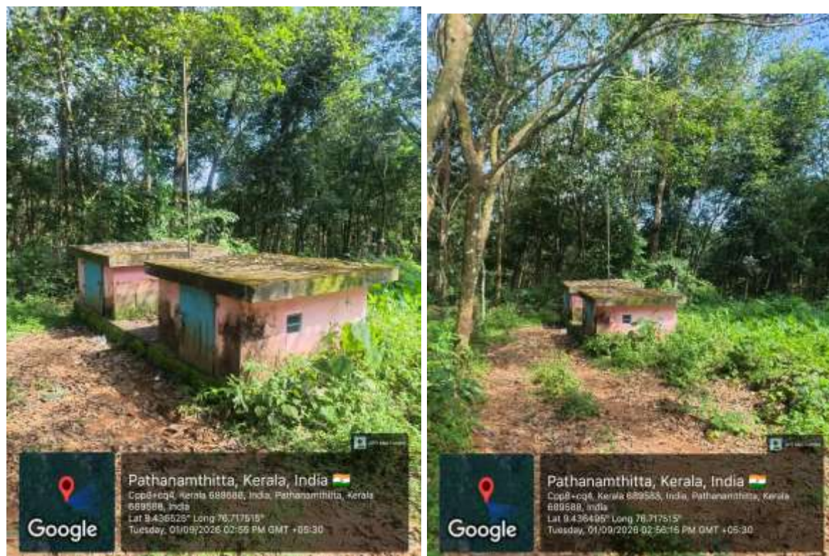
Figure 6: Photograph showing the magazines
